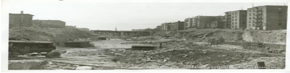
Figure 1: Trench in the Middle of East Tremont
